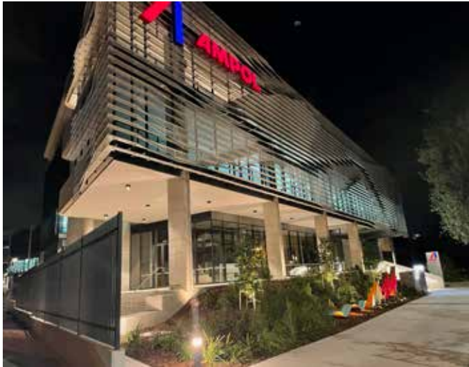
29-33 Bourke Road, Alexandria
