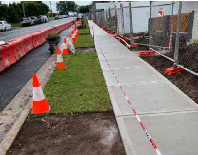
Somerset Road, Narallen - Stage 2
