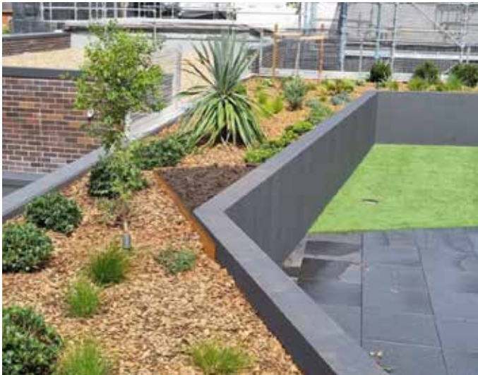
Somerset Road, Narallen - Stage 2
